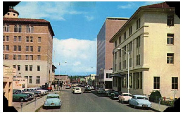
Above is an historic photo from 50 years ago shows the Post Office Building, the Federal Office Building and with the Federal Court Building on Gold Avenue when all three building boiler systems were served by a central mechanical heating and cooling plant.
